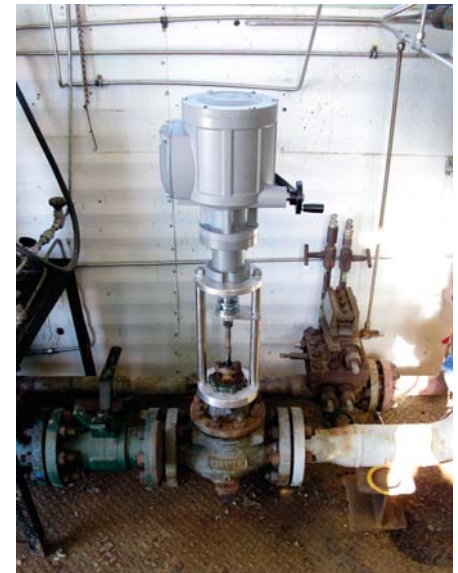
Bear BA-15L Solar Ready Electric Actuator installed
