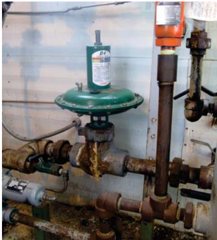
Fisher Pneumatic Actuator powered with methane gas
