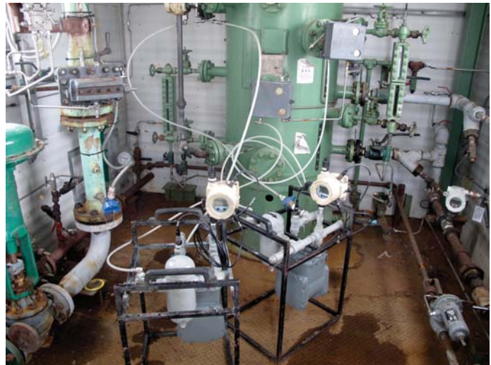
Two Calscan Hawk 9000 vent gas meters measuring the vent rate of the pneumatic controls and actuators
