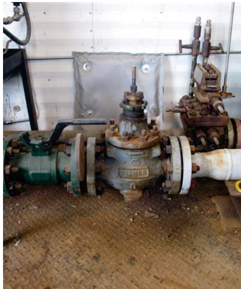
Fisher 3 inch E-Body Valve with pneumatic actuator removed
