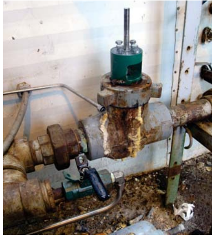
Fisher 2 inch D Body Control Valve with pneumatic actuator removed
