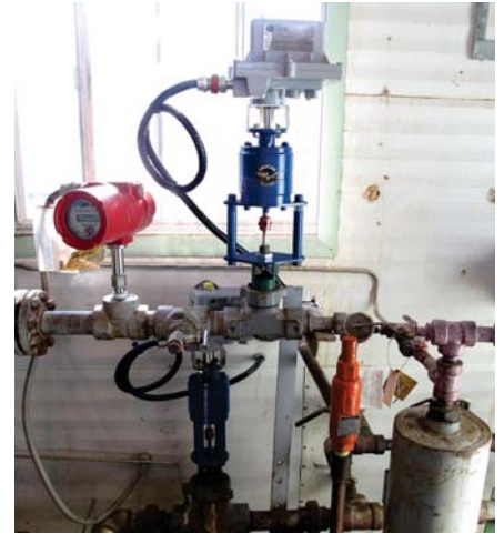
Bear SA Solar Ready Electric Actuators installed on D Body Control Valves
