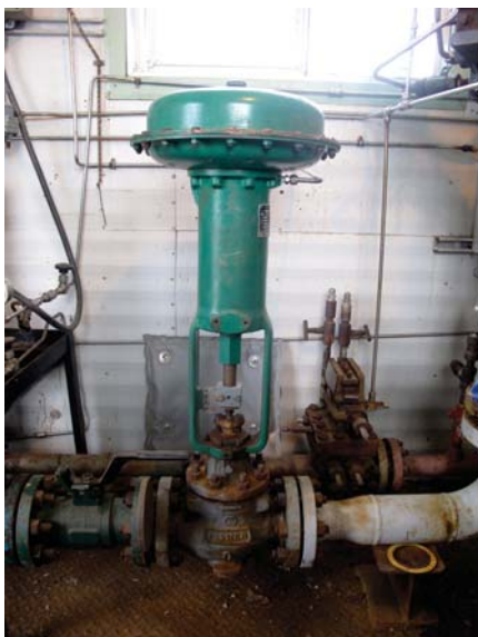
Fisher 667 Pneumatic Actuator powered with methane gas
