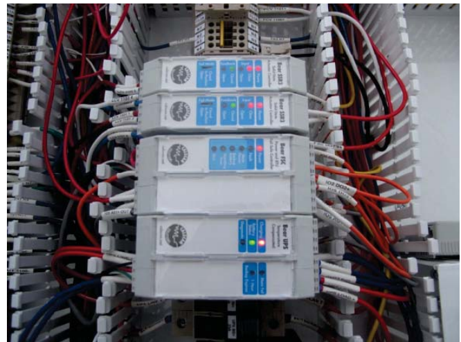
The Bear Failsafe System is Designed and Manufactured in Alberta by Calscan and is Div2/Zone2 Certified from -40°C to 50°C
